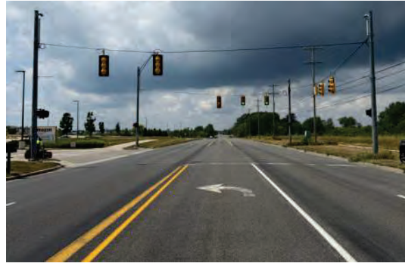
Westbound 68th Street approaching East Driveway
